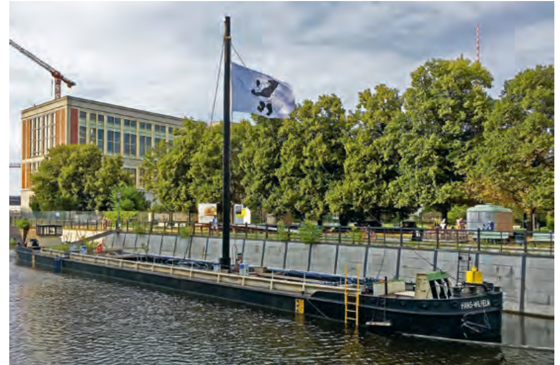
Test filter on the “Hans-Wilhelm”, a barge set up in the Spree Canal near the Flussbad Garden cc 2018 Martin Henseleer
